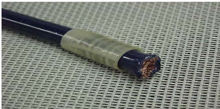
Photo 8: Z-Block tape wrapped around cable
