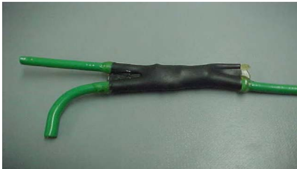
Photo 14: Typical three legged crimp splice with PRT squeezed flat
