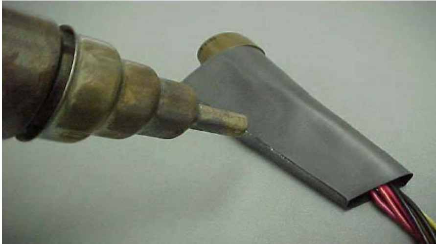
Photo 2: Shrinking tubing using a reducer nozzle.
