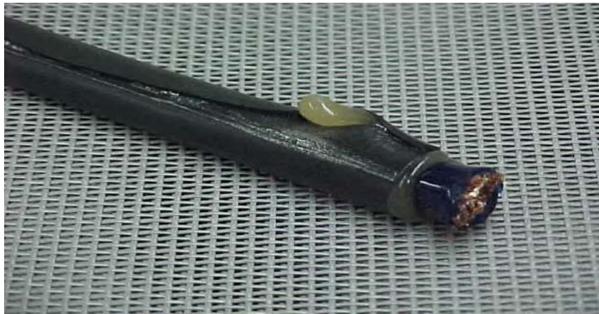
Photo 7: Typical overlap seam rupture
