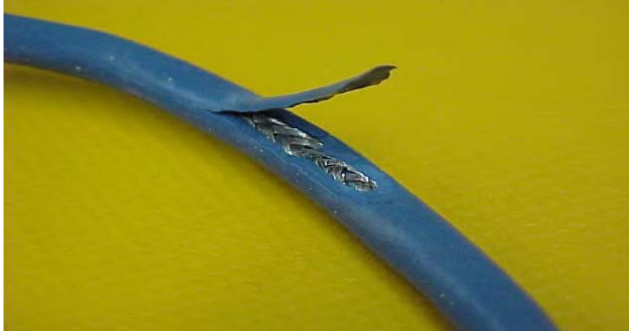
Photo 2: Typical cable jacket damage.
